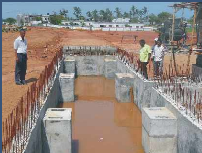
Work going on at the Gopalpur Port site
